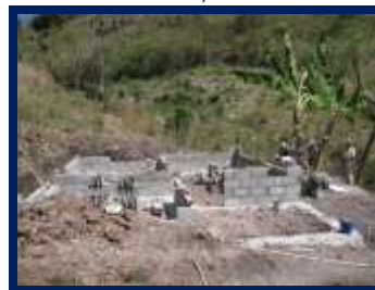
Building up the walls
